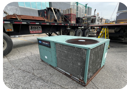
Old HVAC Unit
